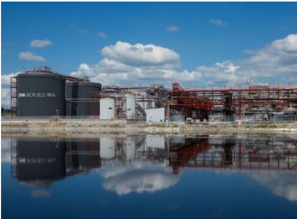
Photo 15 UPM's Lappeenranta biorefinery plant
