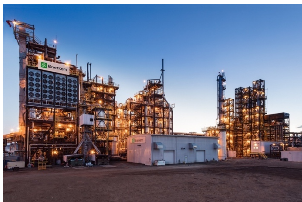
Photo 7 The ENERKEM plant at Edmonton, Alberta, Canada
