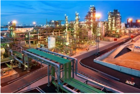
Photo 13 NESTE's HVO plant in Rotterdam
