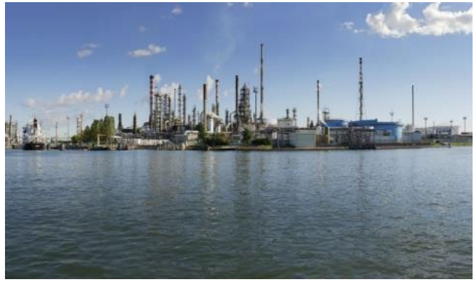
Photo 14 ENI's Green Refinery plant in Venice
