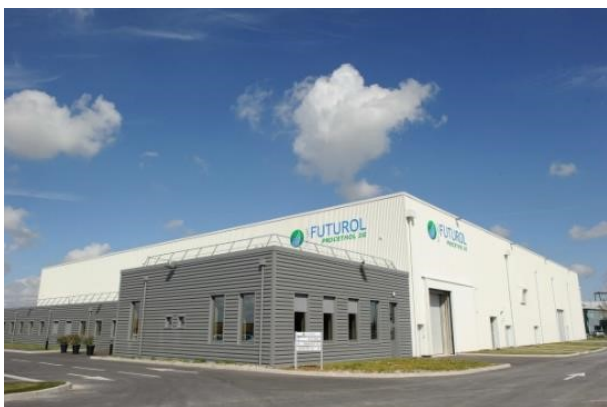
Photo 5 The FUTUROL pilot plant at Pomacle, FR
